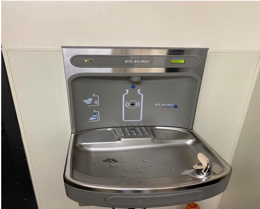
Elkay water filter / fountain combo. Will also fill reusable water bottles. Replaces 5-gallon bottle dispenser.
